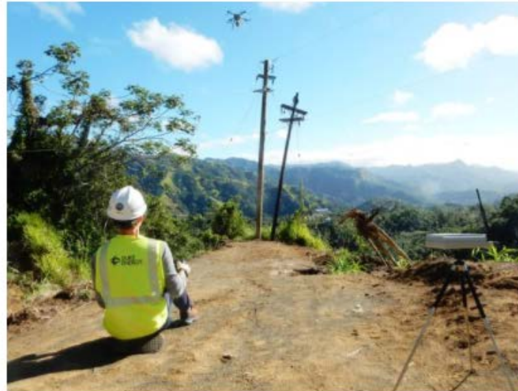
The North Carolina-based company Duke Energy is using five drones to find and restore downed power lines in Puerto Rico. DUKE ENERGY
