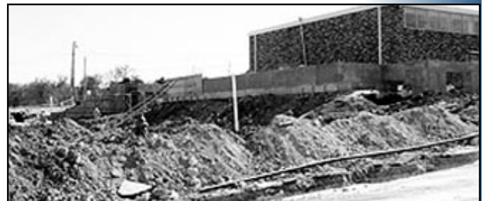
Construction on an addition to the Administration Building is underway.
